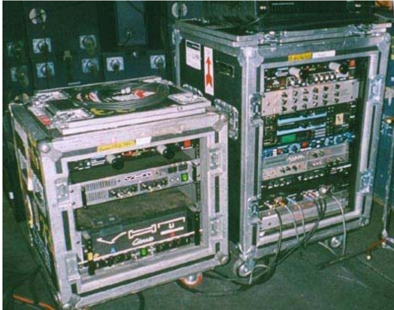
Amps and effects racks.
